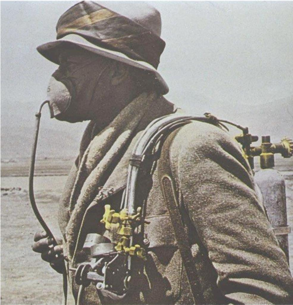
*The oxygen apparatus of the 1920s: a light duralumin frame on the back carried four oxygen cylinders of a total weight of about 20 kilos. The oxygen, bottled at 120 atmospheres, was released through valves, and the air supply was controlled by way of flow-meters which were in front of the climber. Four oxygen cylinders supplied enough gas for approximately five hours. Empty cylinders could be replaced by reserve cylinders.*
